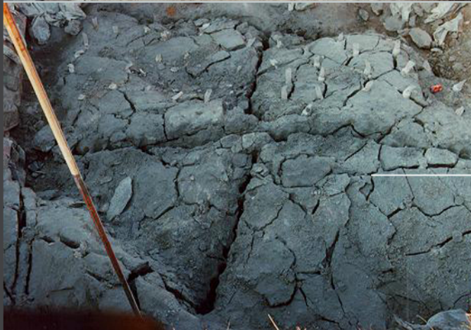
Good cross cracking.
