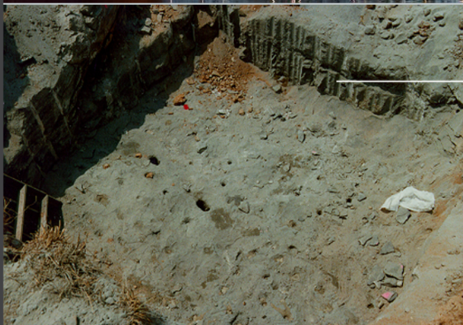
Drill pattern and wall channeling.
