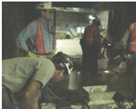
Drilling into volcanic rock that has cavities from gas pockets, pumping mortar into holes
