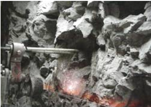
Drilling into volcanic rock that has cavities from gas pockets, pumping mortar into holes
