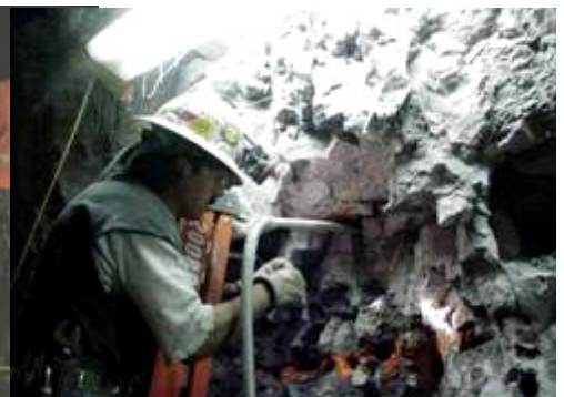
Drilling into volcanic rock that has cavities from gas pockets, pumping mortar into holes
