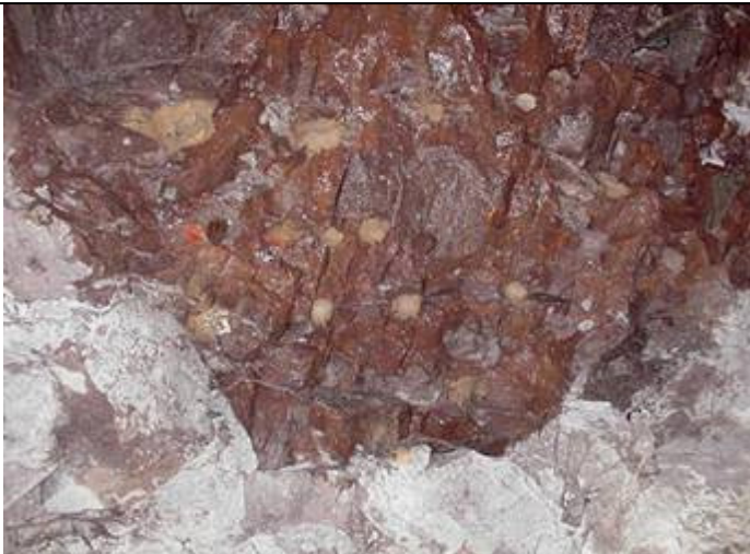
Cracking caused by Rock Splitting Mortar note how gas pocket was filled
