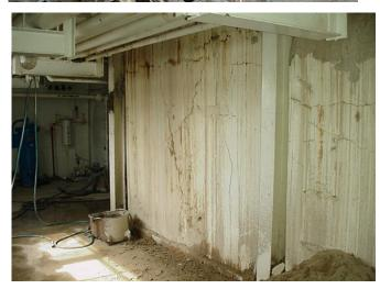
View above left of compressor before removal, drilling inside with Track Drill using water for dust control. Middle left looking down on drill and foundation which was 24 x 19 feet. Above, cracking starting and left, cracking on foundation as seen from basement.
