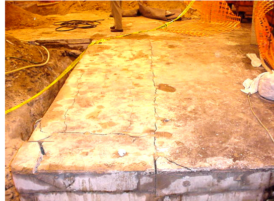
Daigh "pre-split" foundation so only half of it had to be removed.
