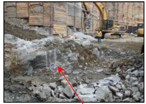
Problem Rock Excavated. Note clean cut Da-mite used for tiebacks
