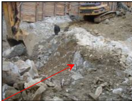
Rock was dug with an excavator and a mechanical hammer
