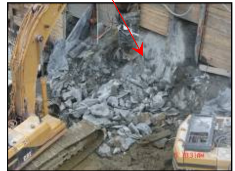
Problem Rock Excavated. Note clean cut Da-mite used for tiebacks
