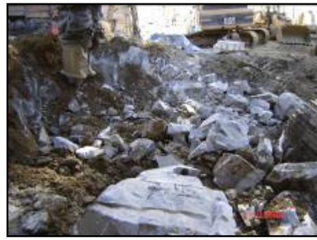
Rock was dug with an excavator and a mechanical hammer
