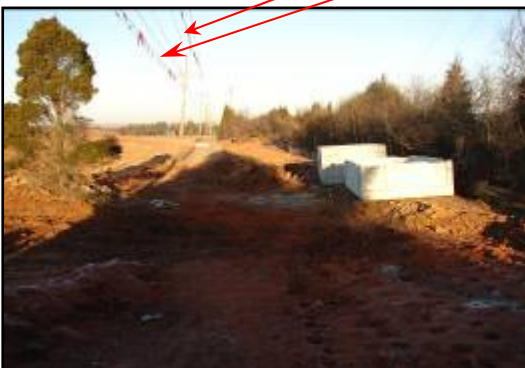
Two manholes next to power lines 13ft x21ft x18ft
