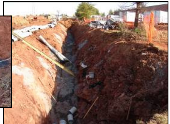
Preparing to lay pipe in trench
