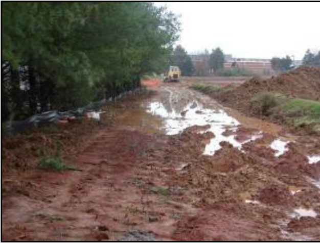
Trench to be drilled alongside the duct bank
