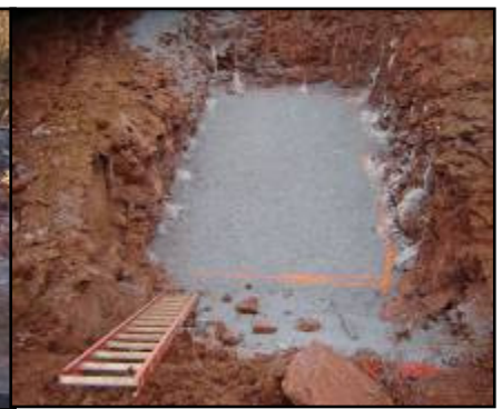
Manhole pit after excavation
