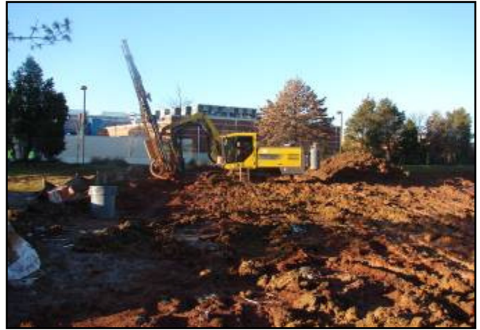
Drilling 2 1/2" holes through 5 feet of overburden
