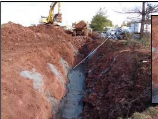
Digging Trench with 325
