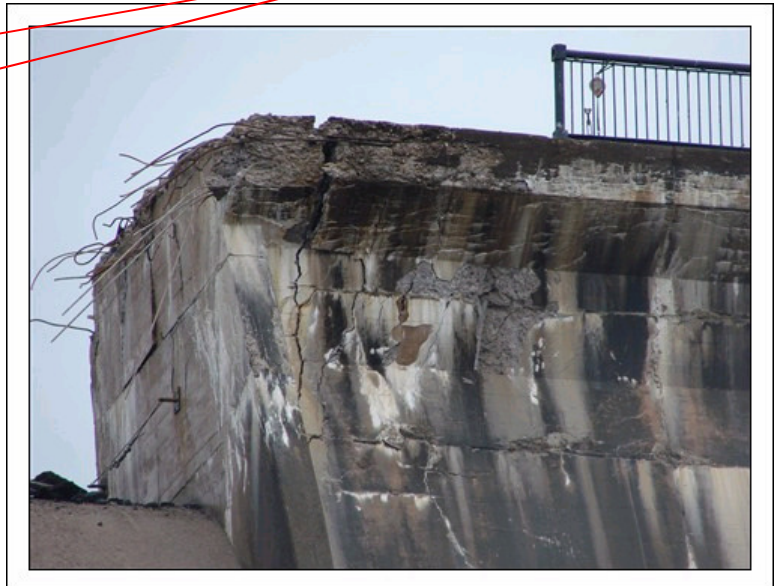
Initial Cracking
