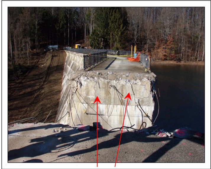
Initial Cracking
