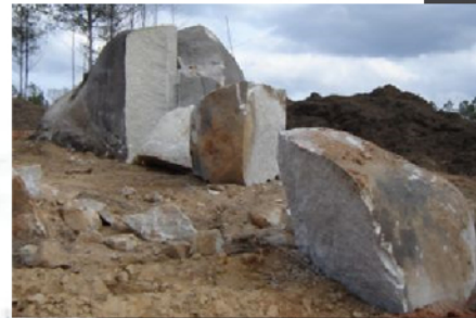
Boulder is broken into movable pieces.
