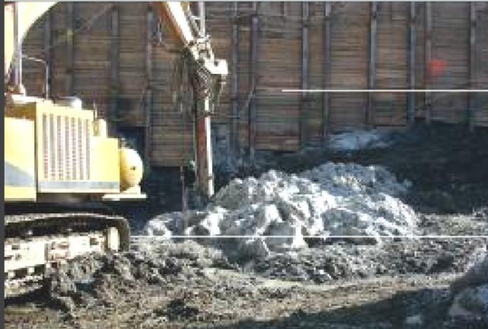
Da-mite was also used on the wall to excavate rock so that tiebacks could be placed.
