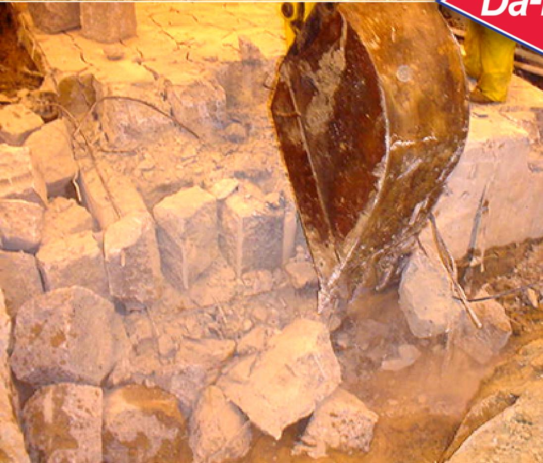
Digging fractured foundation with loader backhoe.
