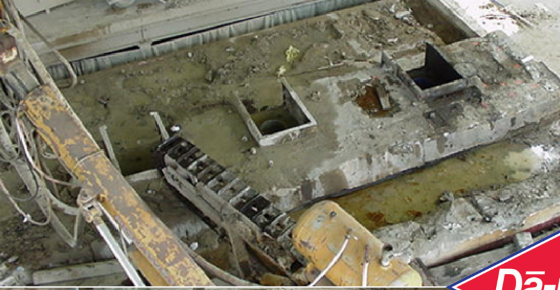
View from above: Drill & Foundation 24' x 19'
