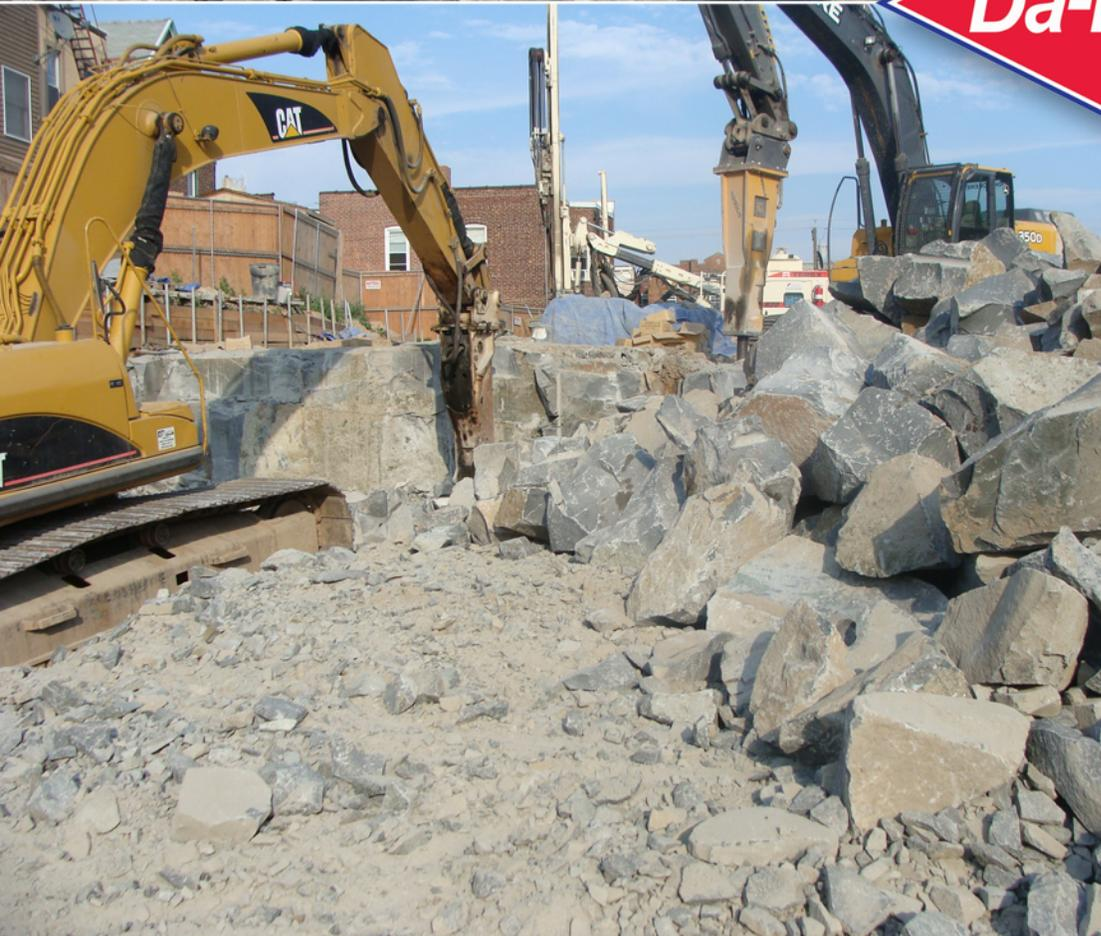
Impact hammers could not break the rock. Da-mite was required to create initial cracks so the hammers could be effective.
