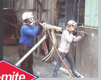
Drilling holes the day before shutdown with "jack leg" drill while equipment is still running.
