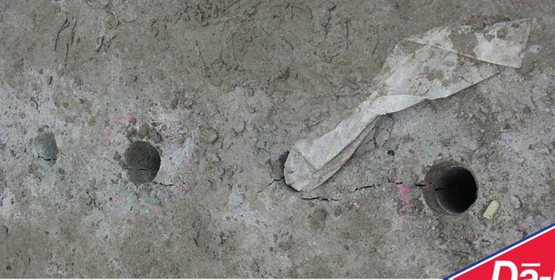
Cracking occurred from hole to hole full depth.
