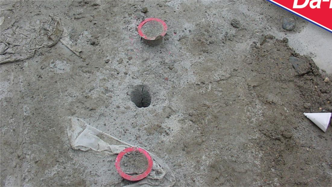
Da-mite was loaded in sleeved holes due to wet conditions in the holes.
