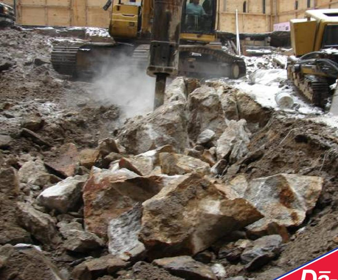
Cracks were large enough to allow Hammer to separate the rock and create "chunks" of rock.
