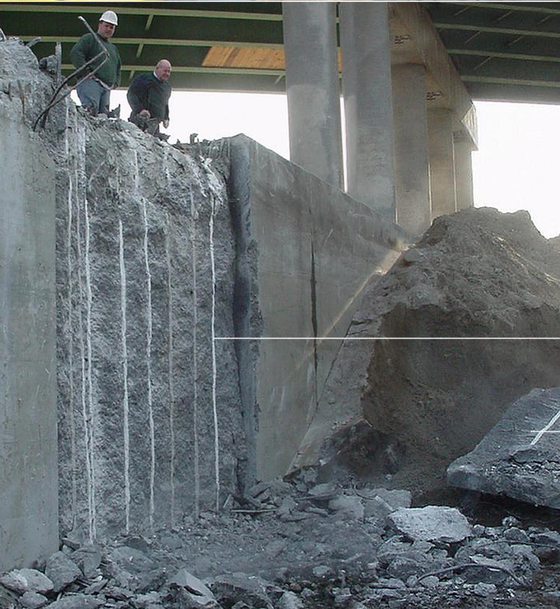
Concrete broke along lines of holes.
